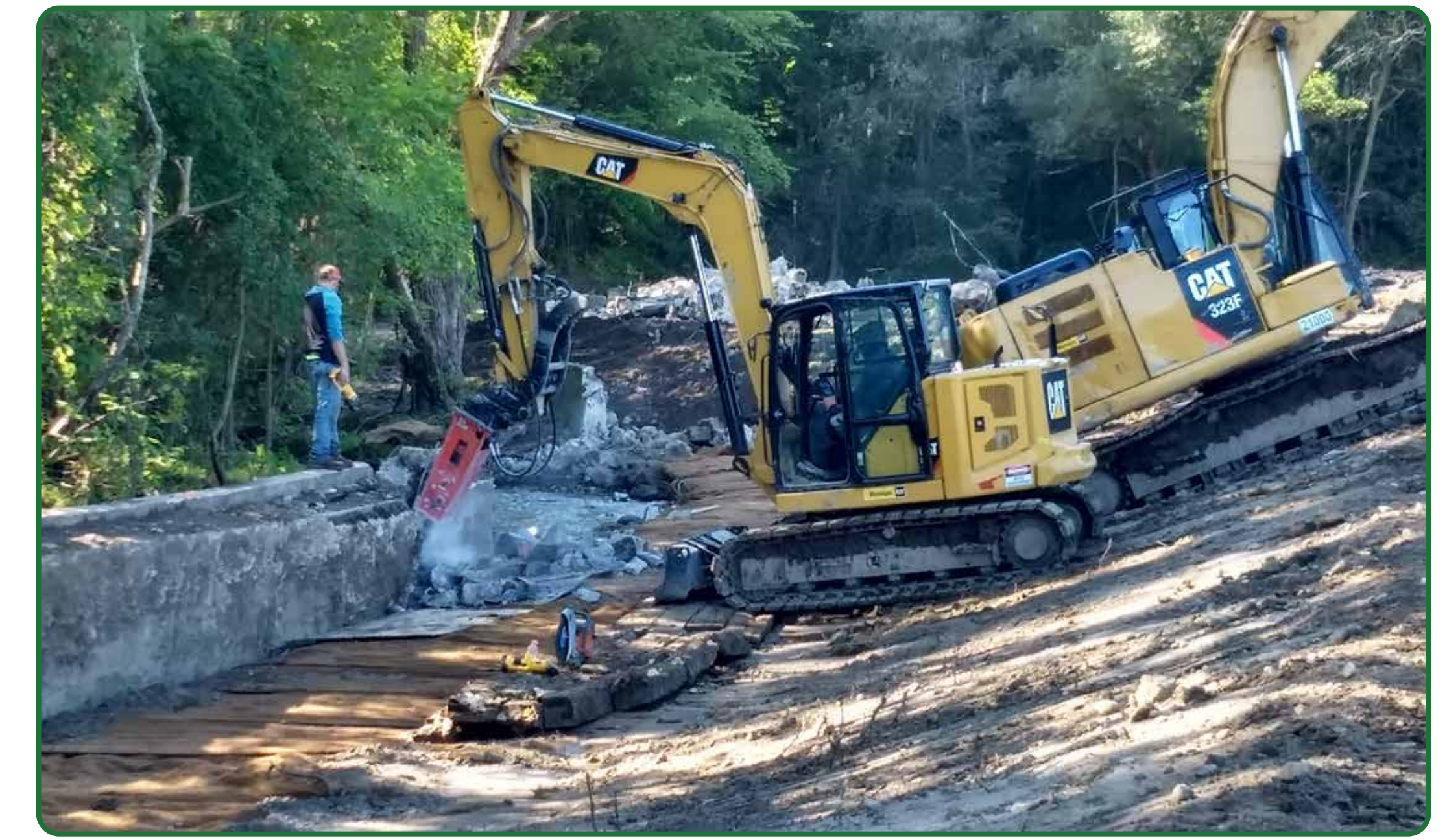
Removal of concrete wall
