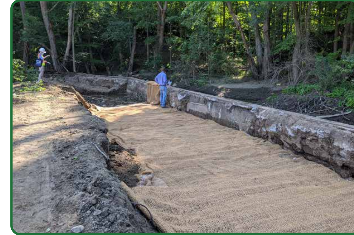
Inspection of brush layering separation blanket
