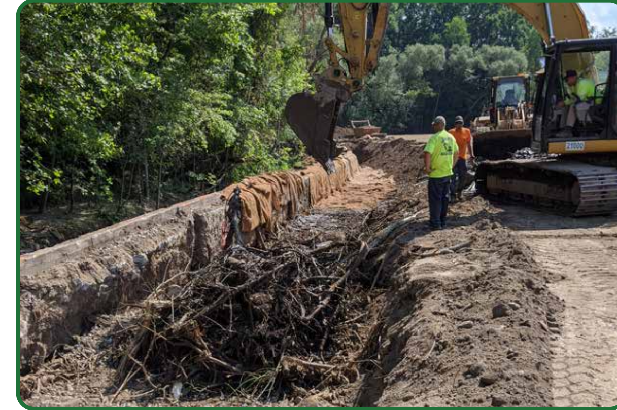
Installation of brush layering
