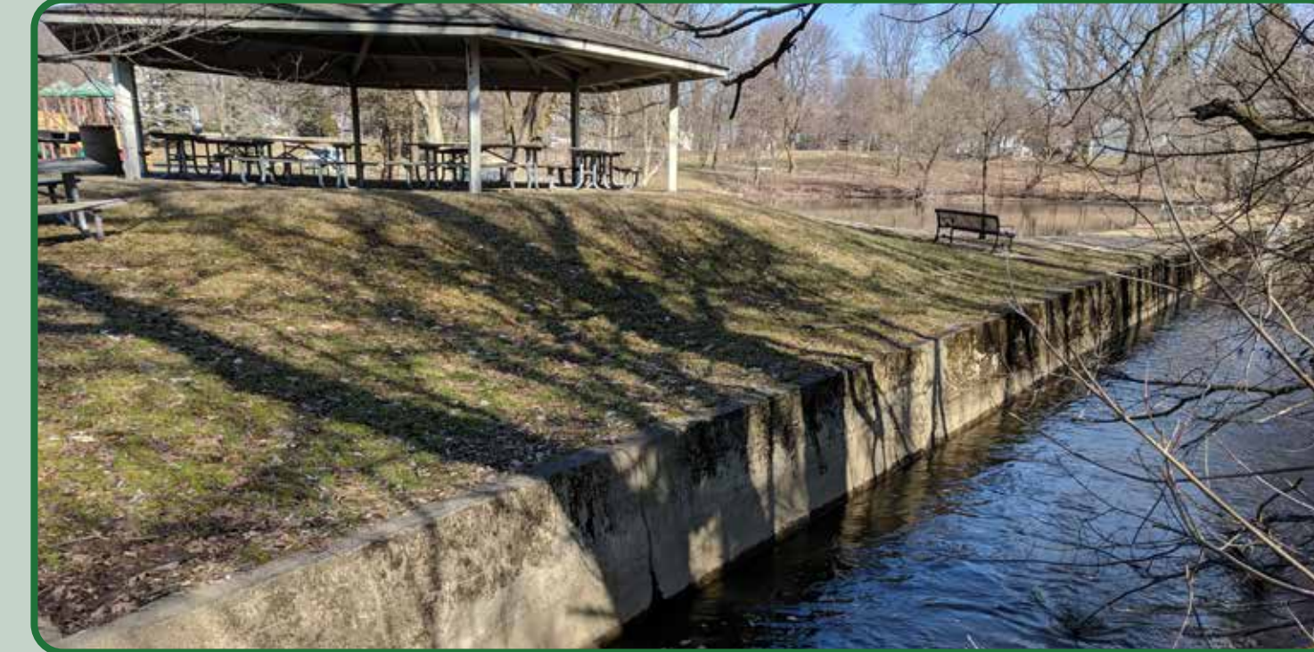
Concrete wall channelizing creek
